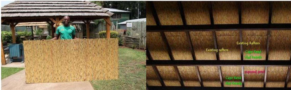
Standard Cape Reed Ceiling-board 1.2m (4') by 2.4m (8') Cape Reed Ceiling-boards fitted to and existing truss system
